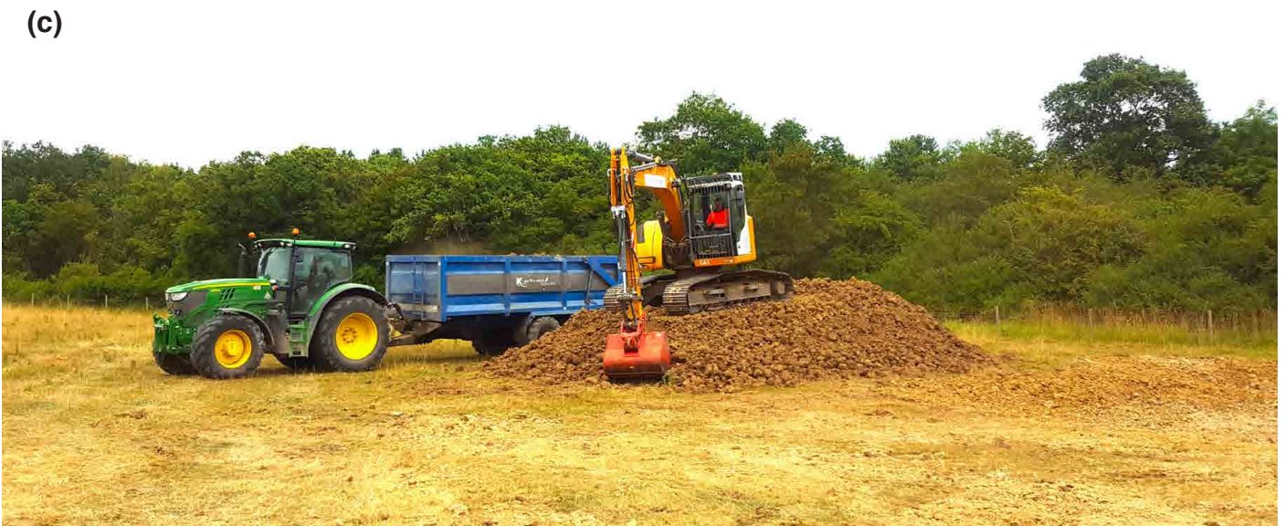
(c) Medium sized ponds of 200-500 m 2 can be excavated using 15 tonne machines. Larger ponds are more efficiently created with larger machines.
